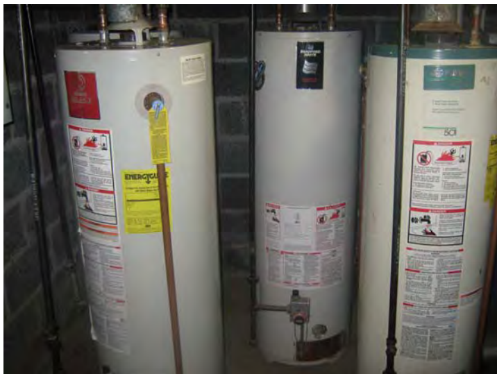
View of gas fired hot water heaters – 1 natural gas-fired domestic hot water tank per unit.
