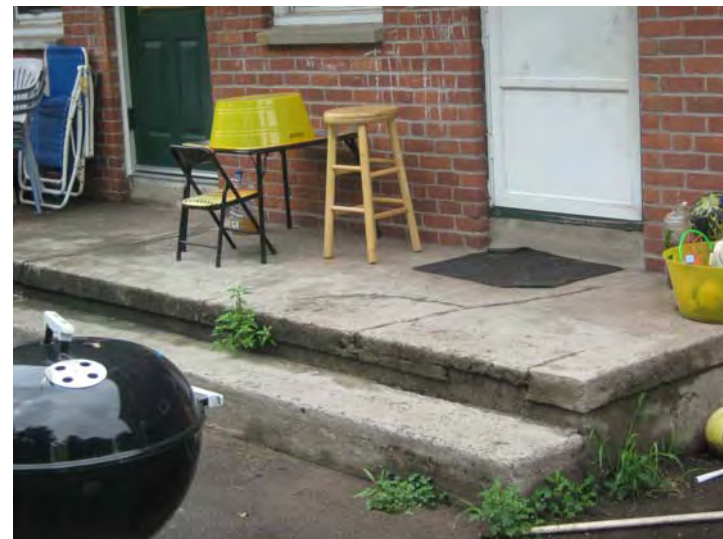
Areas of cracking and spalled concrete noted at the concrete stoops.
