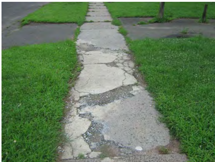
Areas of cracking and spalled concrete noted at the concrete sidewalks.
