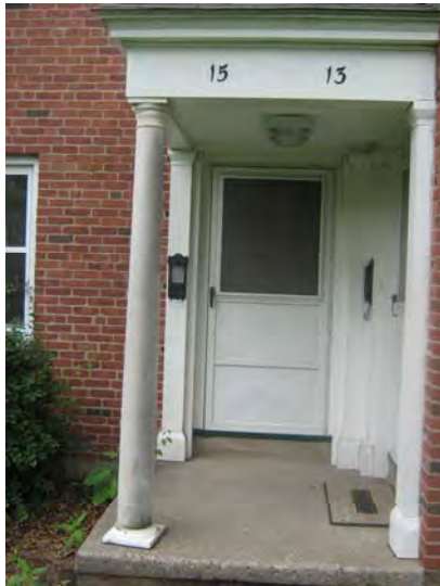
View of support column at entrance canopy exhibiting displacement.
