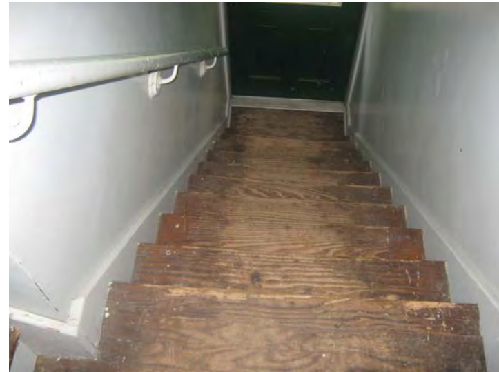
View of aged and deteriorated wood flooring in common stairway.
