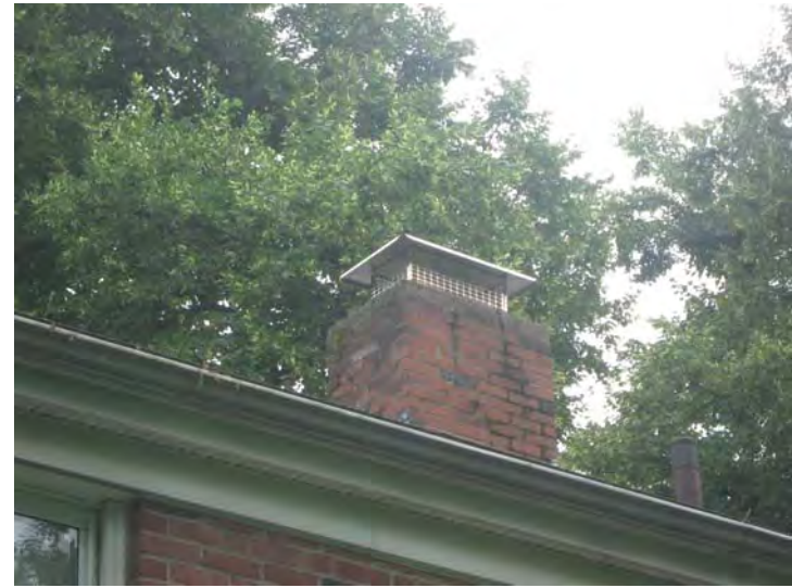
Cracked and spalled brickwork as well as deteriorated mortar joints noted at chimneys.
