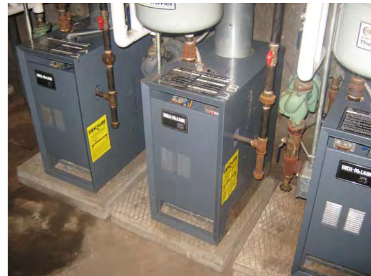
Weil-McLain boilers for production of hydronic heat – 1 natural gas-fired boiler per unit.
