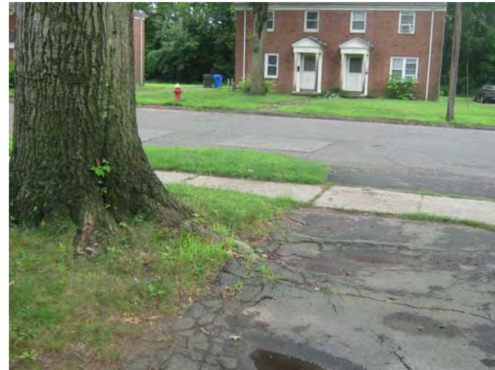
View of cracking within asphalt pavements.
