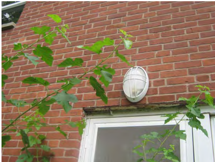
View of surface corrosion on steel lintel.
