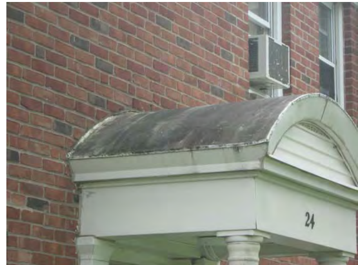
View of weathered/deteriorated roof covering at entrance canopy.
